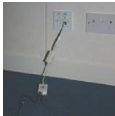
Connect microfilter to BT phone outlet.
